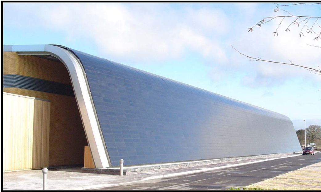
Building-integrated CIGS, 85kW Shell Solar
